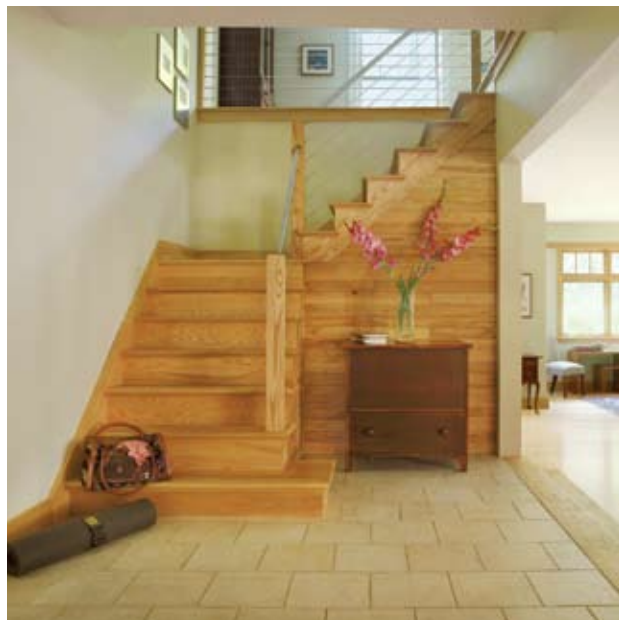
Above: Heaton and her husband updated the kitchen with skylights, new cabinets and countertops, and an island with a four-inch maple surface. Right: Stainless steel handrails and cables add a contemporary element to the staircase. The wood floors at right are Vermont brown maple; the stairs and trim are native ash.
